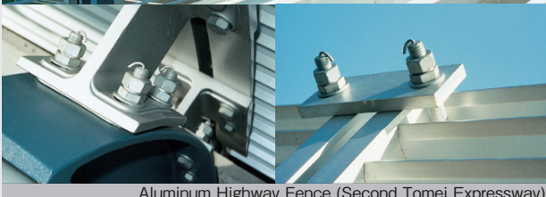
Aluminum Highway Fence (Second Tomei Expressway)
