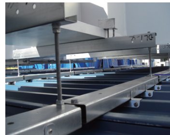
◀ Pier Cover Plate Mounting
