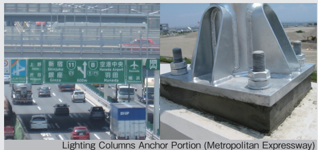
Lighting Columns Anchor Portion (Metropolitan Expressway)
