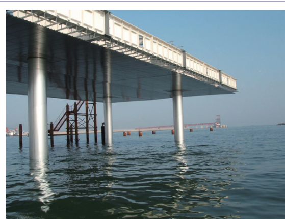
◀ Pier Cover Plate Mounting
