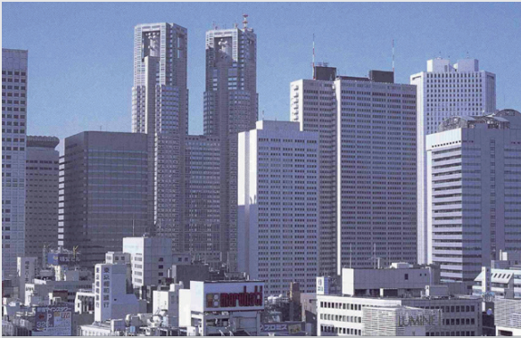
High-Rise Building Exterior Wall & Curtain Wall
